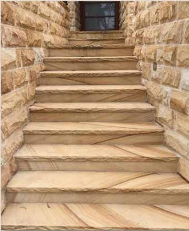
TEAK STONE STAIRCASE STEPS
